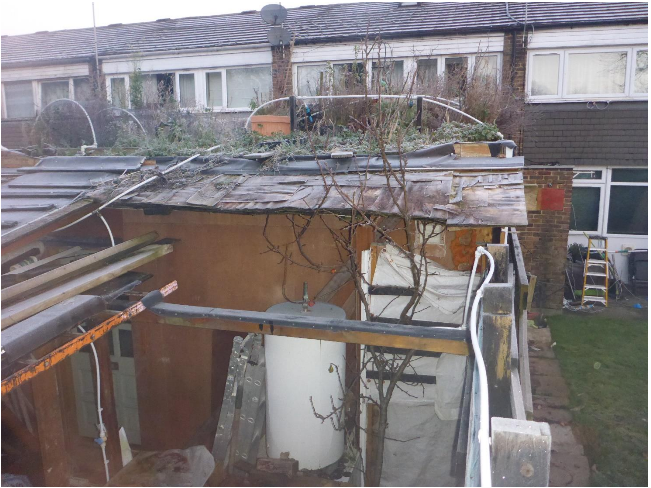
Rear Extension and Terrace Removal 22 1 20
