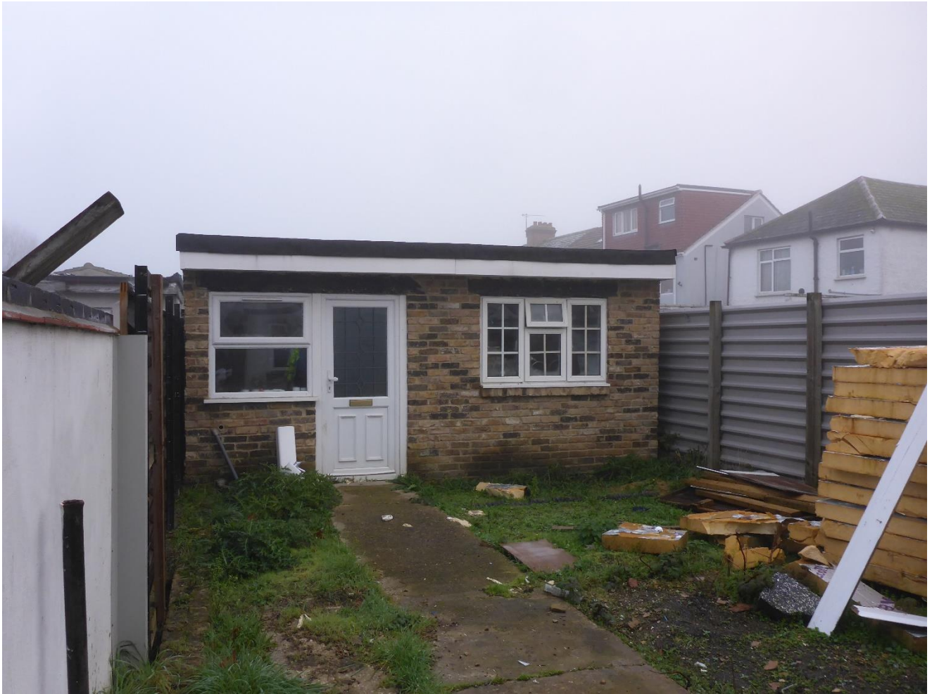
Shed for Bed Removal 30 November 2019
